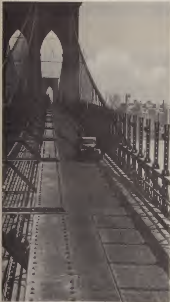
Brooklyn Bridge, before the heightened trusses along the outer edges were completed—note section immediately right of tower.
